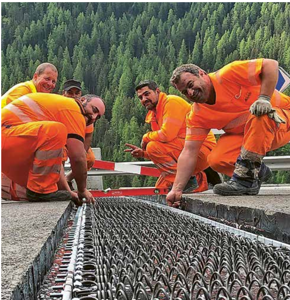
The continuous training of our employees ensures professional processing. Reports comprehensively document our services as part of quality management in accordance with ISO 9001.
